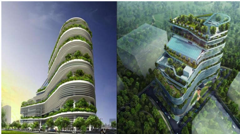
Figure 5 Solaris Building, Singapore
